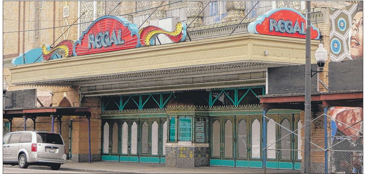
We Are Our Brother's Keeper secured a grant to restore the New Regal Theater on Chicago's South Side, money that federal investigators say was misappropriated. | FILE PHOTO
